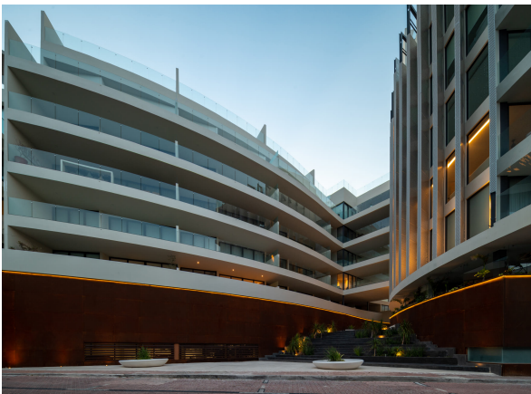
MARILA facade · photograph 30
