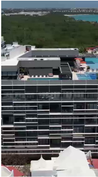
Real drone footage · construction progress · v33.jpg
